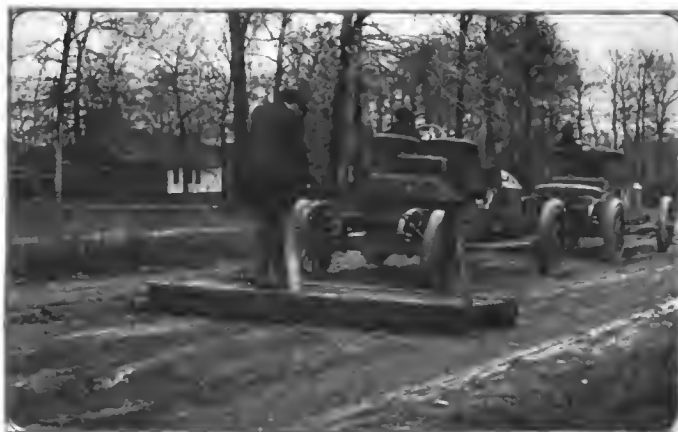
Two Premier test cars pulling a King road drag over Indiana roads injured by the recent flood
